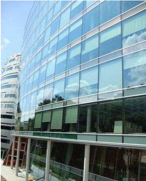
Fig. 1. The architectural example of frontage building with glass windows
